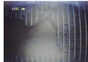
Side View - showing not well-developed SS Screen Section at 207.4 mbgs
